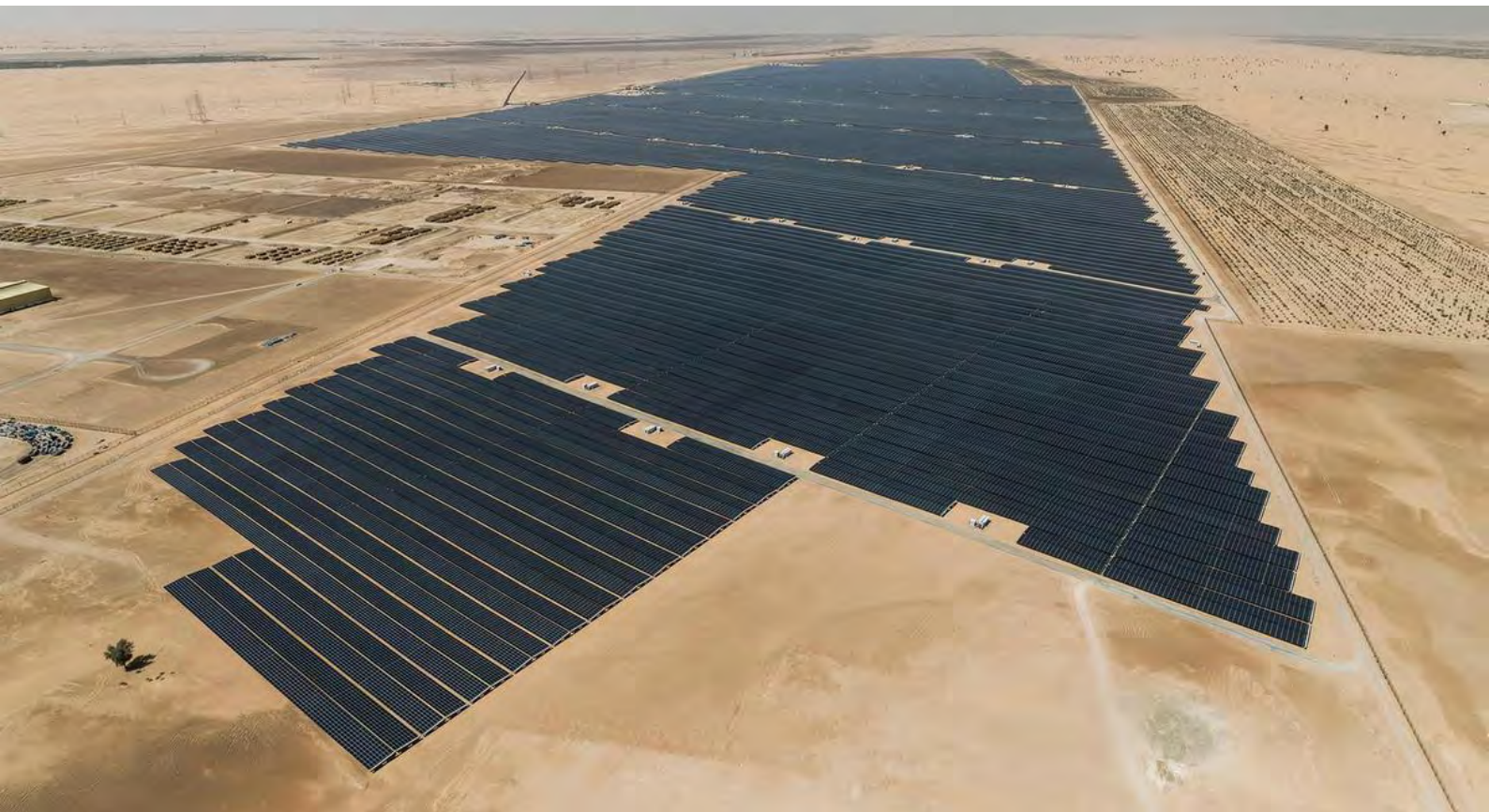
Noor Abu Dhabi solar plant, UAE
